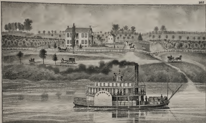
MONTEBELLO FARM. RESIDENCE OF C. F. DARNALL, SEC 18, MONTEBELLO TP, HANCOCK CO, ILL. LAST FOR DOMESTIC SEWING MACHINE
